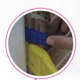
**STEP 6** To hold the door in place temporarily whilst you level it, loosely pack out the jambs. Keep checking they are level as you go along, as this will help to avoid any potential issues in later steps.
