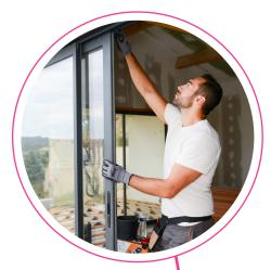
**STEP 15** Check the finished doors to make sure the operation is perfect. The rolling mechanism should be smooth, & all the seals should be weather tight.
