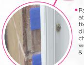
Packers must be used at either side of each fixing to help prevent distortion. Continue to check for any bows, as well as for plumbness & squareness.
