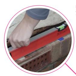
**STEP 1** Use a spirit level & a string line to assess the level of the threshold you are working from.
