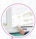
**STEP 13** Once the glass is in place, the beading can be replaced, starting with the shortest piece first. Use a plastic mallet to tap each piece into place. We recommend starting in the corners, & working towards the middle.
