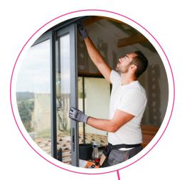
**STEP 16** Check the finished doors to make sure the operation is perfect. The rolling mechanism should be smooth, & all the seals should be weather tight. Make any final adjustments as necessary.
