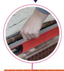
**STEP 1** Use a spirit level & a string line to assess the level of the threshold you are working from.
