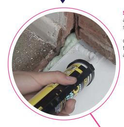
**STEP 6** Run a bead of silicone along the outer edges of each side of the cill.
