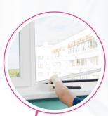
**STEP 14** Once the glass is in place, the beading can be replaced, starting with the shortest piece first. Use a plastic mallet to tap each piece into place. We recommend starting in the corners, & working towards the middle
