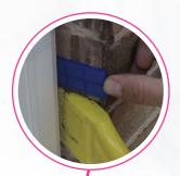
**STEP 8** To hold the door in place temporarily whilst you level it, loosely pack out the jambs. Keep checking they are level as you go along, as this will help to avoid any potential issues in later steps.
