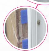
**STEP 9** With the packers in place, fix both outer jambs in place with appropriate fixings.
