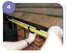
\* Mark the position of the fascia brackets, spacing them no more than 800mm apart (600mm in areas of heavy snowfall) and no more than 150mm from any angle or stopend.
