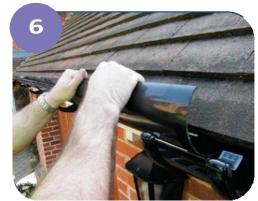
\* Starting at the outlet, fit the first length of gutter using the 'back to front' rule (see below).
