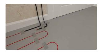
The cold tail joint can be secured in place by taping the cable either side of the joint, a small piece on the heating cable and a small piece on the cold tail. This will ensure the joint is NOT covered with tape.
