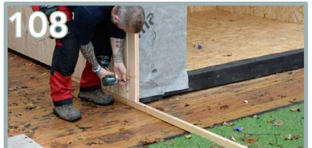
The batten and the T&G board will overhang at the front, as indicated on the layout shown above. Pre-drill ready, as these 3 x 80mm screws will go into the front panel.
