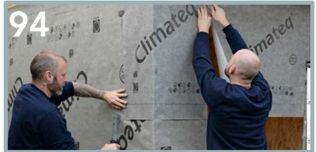
Staple into place and remove the excess from the door section.
