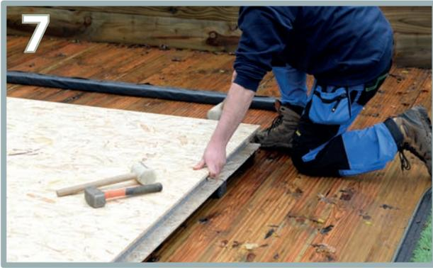
Using a rubber mallet, knock the second panel into the first for a tight fit.
