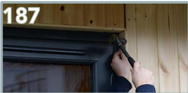
Secure into place with 5 x 30mm nails. Repeat the process for the opposite side of the door frame. Then repeat the same application around the window frame.
