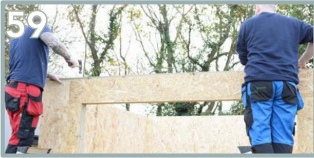
59 Insert the front wall plate (AL), knocking into place. Expect this to be tight fitting. Ensure it is flush to the top and ends.
