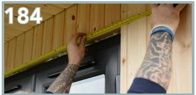
If any of the boards are slightly oversized, you will need to measure out your required length. Start with the top board.
