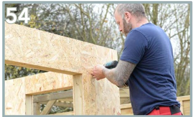
54 Position the screws on the Lintels OSB and screw into the wall batten behind. Secure into place using 4 x 35mm screws internally and externally, 2 x 35mm screws each side of the lintel insert.
