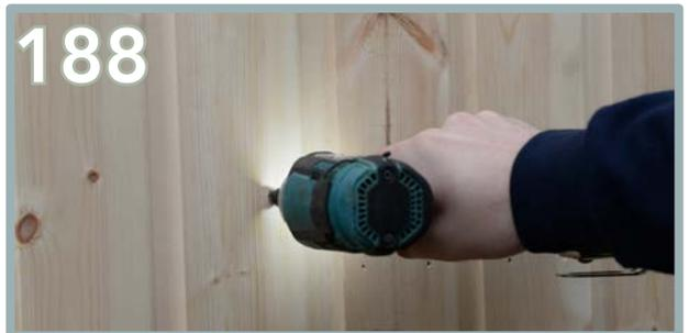
You will need to fill in the holes of each screw in the T&G panels to create a flat finish. Further countersink the screws, and enlarge the hole by 10mm.
