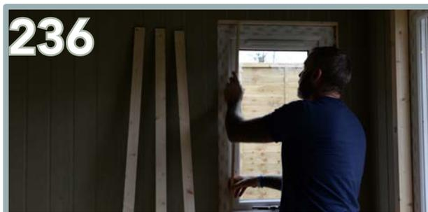
Apply the side framing, using 5 x 30mm nails per board.
