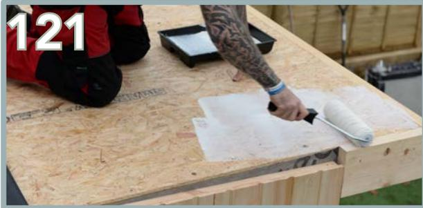
Pour the glue into a paint tray and use a roller for easier application.
