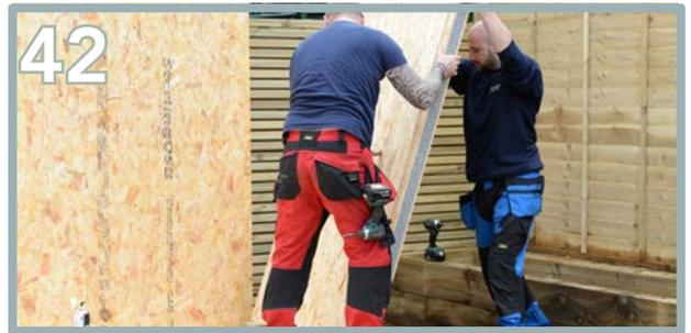
42 Repeat the same process for the right hand corner (G). Add foam and knock into place. Ensure the panel is flush to all edges as mentioned and shown above.
