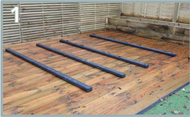
Lay the bearers down and spread them out roughly ready to position the floor panels on top.
