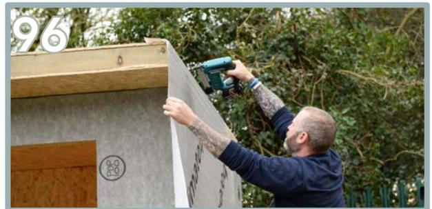
Fold onto the roof, stapling into place.
