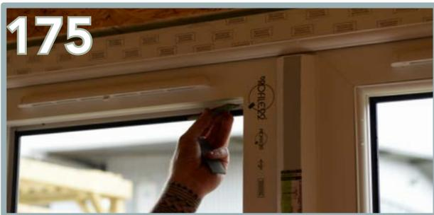
Apply silicone and stick the packers at diagonal opposing corners. Place the pane into position, ensuring it is centralised and packed correctly, holding the pane square.
