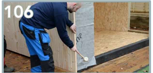
Apply the next side panel (BA). Softly knock the second side panel into the first, so the T&G interlocks the panels together. Use a rubber mallet for a softer application.
