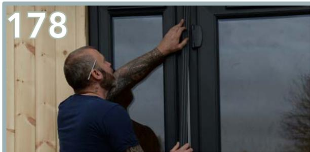
For the adjoining frames, attach the strip provided with the metal capping. This will clip into the fixed metal capping. To further secure, you can also add glue to the strip.
