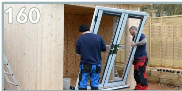
Lift and angle the frame and sit into the ledge. Butt up against the wall panel.
