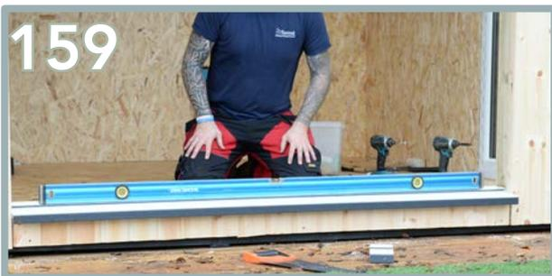
Place the ledge onto the silicone. Ensure it is level and the back edge meets the first edge of the back OSB sheet (The same positioning as the window).
