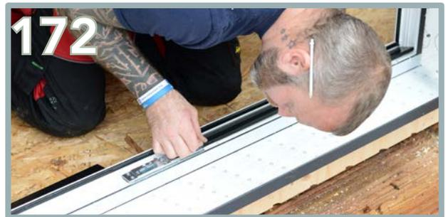
Clip the plastic strips back into the door frame to hide the screws.
