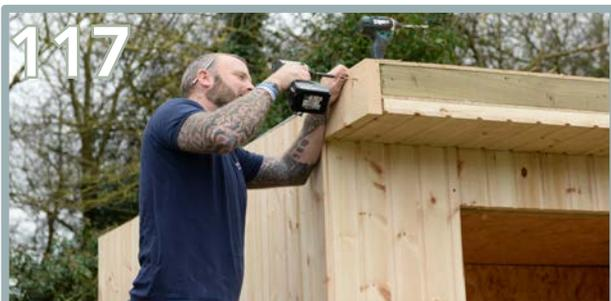
Using 2 x 80mm screws, secure the side fascia. Ensure this is flush to the top and front, whilst butting up against the T&G side panel. Repeat this process for the other side.
