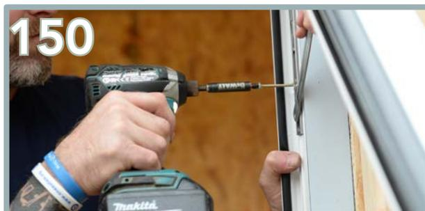
Fix the sides of the frame to the wall panels using the star head 112mm screws at the measurements marked out. Don't forget to fix the top and bottom of the frames.
