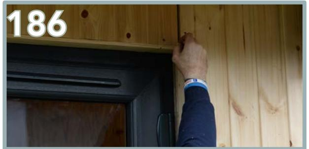
Using 6 x 30mm nails, secure the top board into the lintel. Repeat the same process for trimming the sides.
