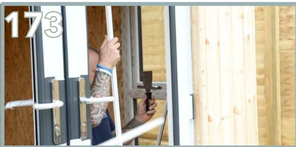
Remove the beading once again around the door, ready to insert the pane.
