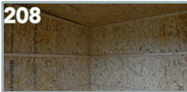
On the left hand side, apply the 45x28mm battens in between the front and back battens. These will flush end to end. Position each batten at the same height as the back.
