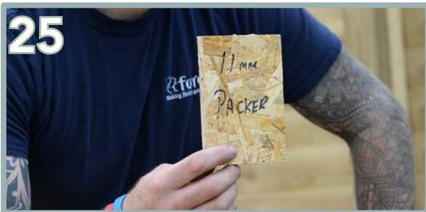
As part of your assembly pack, you will have been provided with an off cut of OSB to use as an 11mm guide when positioning the floor plates.
