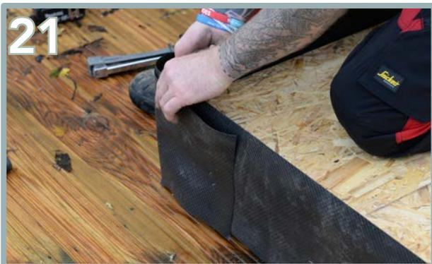
Once fully wrapped around the base, overlap the starting point and staple into place.
