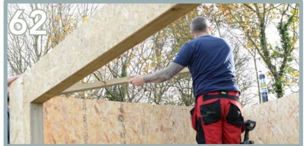
62 Insert the side wall plate (AK). Pre-drill and secure with 4 x 125mm screws. Repeat the process for the other side wall plate and back wall plate with expanding foam and 125mm screws.
