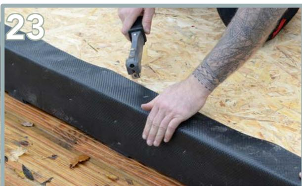
Continue folding the overhang and corners of DPC onto the OSB sheets as you make your way around and staple in place.
