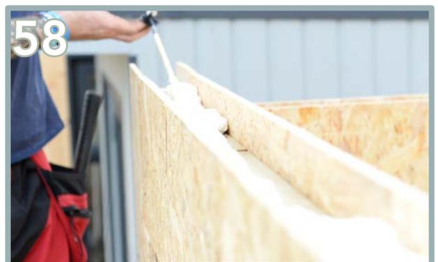
58 Use the expanding foam into the top groove, ready for the wall plates. Start at the front.
