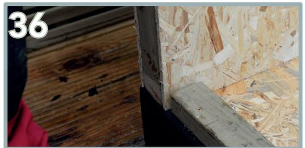
In the left hand corner, the wall panel will be flush to the edge and the floor plate as shown above.
