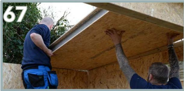
Lift up the first roof panel (V). Ensure at least 2 adults can lift up the roof panels carefully. Measure the overall width for the roof and allow 2mm each side in case of a slight oversize in roof panels.
