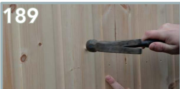
In your fixing box, there will be wood plugs. Insert one at a time, snap off and hammer further into the hole.
