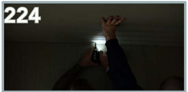
Use 4 x 50mm screws on each side and 2 x 50mm screws in the centre for both panels.
