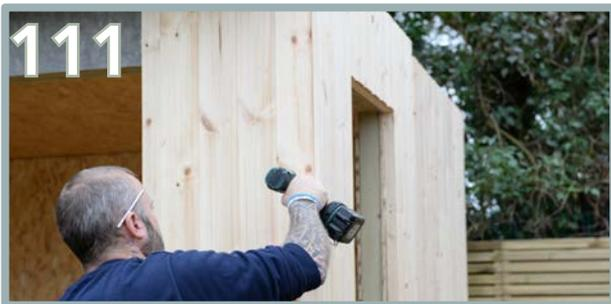
Apply the front panel (AU). Ensure it is butted up against the side panel and flush to the door section. Use 6 x 80mm screws per panel. Ensure you use 3 x 80mm screws down each side of the cladded panel.
