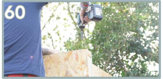
60 Pre-drill and secure with 4 x 125mm screws. Repeat the same process for the back wall plate (AL).
