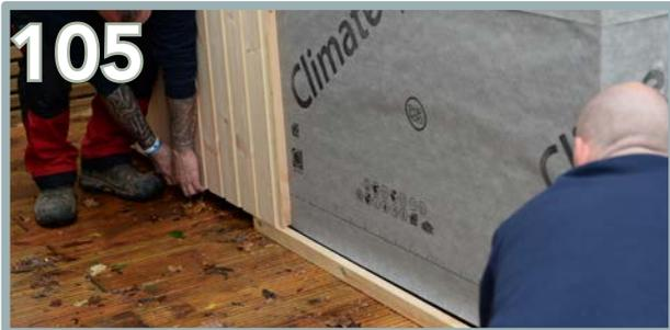
Ensure the cladded panels are 45mm off the ground. If you are using the batten as a guide, slightly lift up the secured panel to ensure it is carefully removed to prevent any damage.
