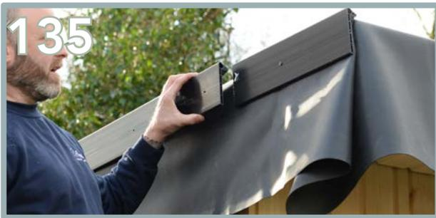
Apply the piece previously cut to size. Ensure it is flush to the front edge and butt up against the plastic trim already pinned into place.
