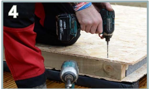
Pre-drill for every process before securing with screws. Pre-drill 5 holes along the edge of the first floor panel. Do not screw in the other side at the moment.
