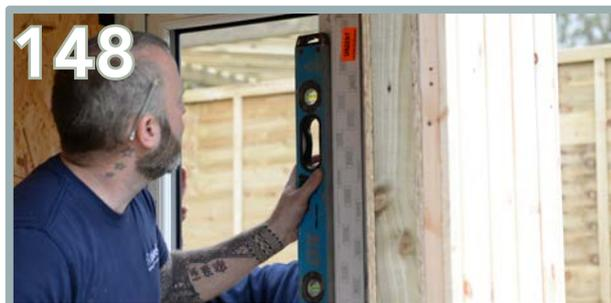
Check that frame is both level and plumb, then drill fixing holes into the frame sides. Pre-drill with a 6.5mm drill bit.
