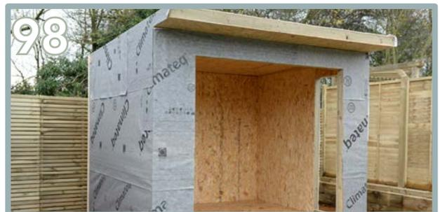
The final result is shown above. You do not need to add membrane to the canopy / the roof overhang.
