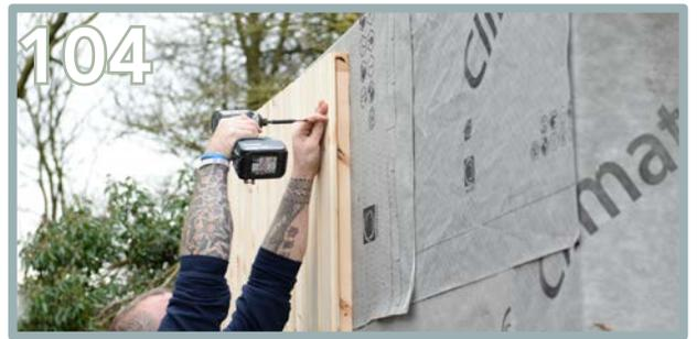
Use 6 x 80mm screws per panel. Ensure you use 3 x 80mm screws down each side of the cladded panel.
