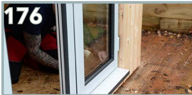
As the pane is positioned, the beading can be installed using a nylon mallet and tapped securely back into place.
