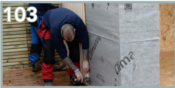
Continue onto the side panels (BB). Knock the first panel in place and ensure it is butted up against the back panel overhang.
