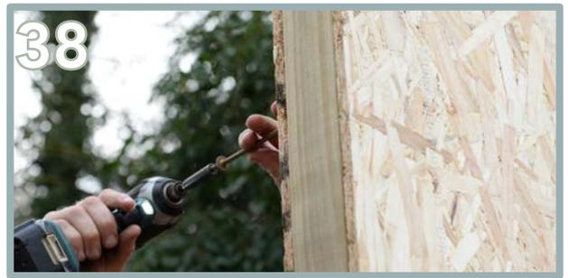
38 Pre-drill and using the star drill bit provided in your fixing box, screw through the back into the side wall panel using 3 x 150mm screws (top, middle and bottom).
