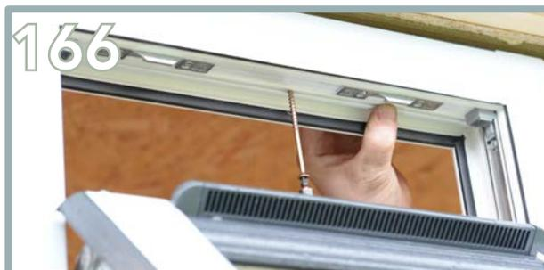
Further secure the window with 1 x 112mm screw into the top and 1 x 112mm into the bottom.
