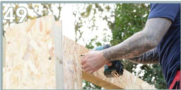
Position the screws on the wall panels OSB and screw into the window insert batten behind. Secure into place using 4 x 35mm screws internally and externally, 2 x 35mm screws each side of the window insert.
