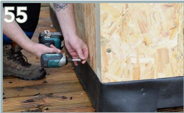
55 Once all of the wall panels are up, begin to secure each wall panel to the floor plate underneath. Use 3 x 35mm per panel externally.
