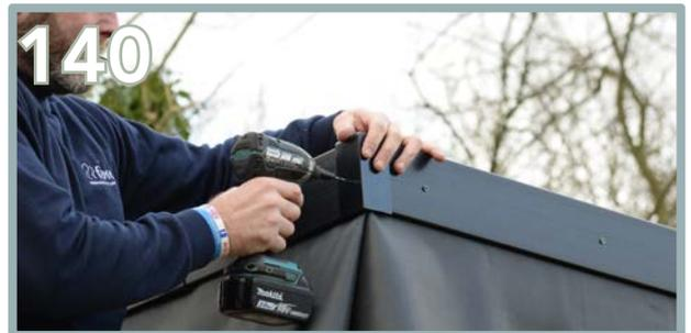
Hook and position onto the corner. Pre-drill to provide a hole for the pin.
