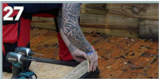
Repeat the process with the front floor plate (AL). Ensure the one end is flush to the side and 11mm from the front edge.
