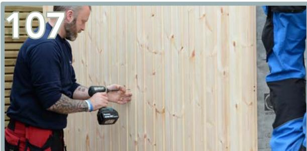
Using 3 x 80mm screws, screw the one side into place.
