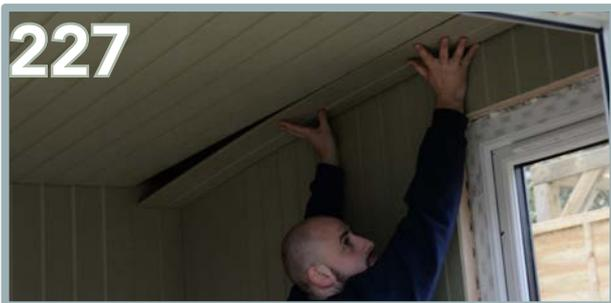
Apply the final and trimmed beaded panel. Use 8 x 50mm screws to secure.
