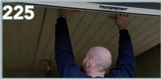
Repeat the same process. Ensure the rounded edge is butted up against the chamfered edge on the first panel.
