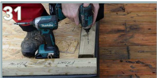
Repeat the process on the other side floor plate (AK) and screw into place.
