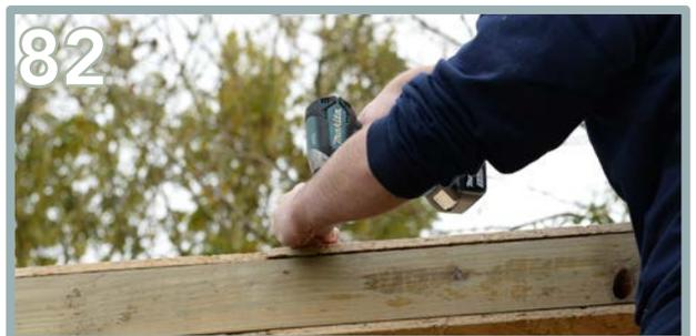
Use 4 x 80mm screws into the panel cap. Use 3 x 35mm screws, in between the 80mm screws to fully secure.
