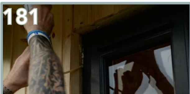
Repeat the application of the expanding foam around the front window and door frame.
