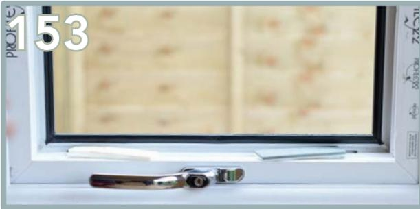
Apply packers with the adhesive silicone. The glass should be packed at diagonally opposing corners to hold the casement square, using the toe and heel process.
