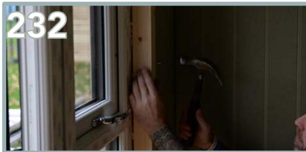
Apply the 45mm boards on top of beaded panel. Ensure this is flush to the inner framing. Use 5 x 30mm nails to secure. Repeat this process on the opposite side.
