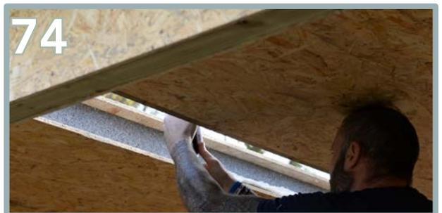
Lift up the second roof panel (U) and apply expanding foam into the inner groove as shown above.
