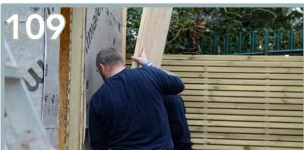
Repeat the same process on the opposite side (BB). Start at the back and butt up against the back panels T&G board. Screw into place.
