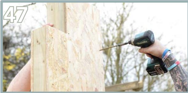
Position the screw roughly 45mm from the outer edge. Pre-drill and screw through the front into the side wall panel using 3 x 150mm screws (top, middle and bottom).
