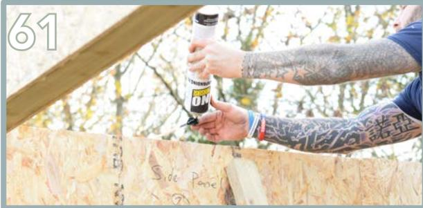
61 Apply expanding foam to the side panels groove.
