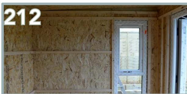
Use 4 x 80mm screws for each of the three smaller battens. You will apply the roof battens on after the beaded wall panels have been installed.
