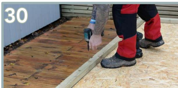
Your side floor plates (AK) will fit in between your front and back plates. Ensure 11mm from the outer edge and 11mm at each end. Once happy with the position, pre-drill and screw into place using 4 x 125mm screws.
