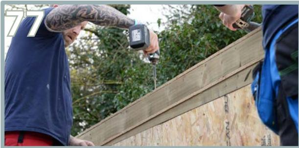
Repeat the same process as the first roof panel using 4 x 150mm screws along the edge to fully secure the roof. Then secure the second roof panels opposite corners with 2 x 150mm screws.
