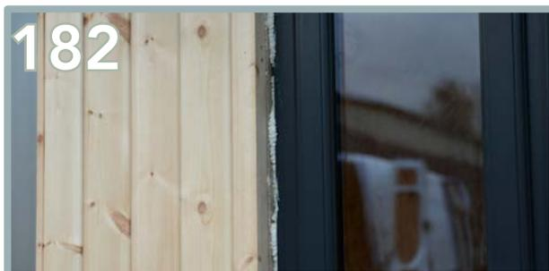
The expanding foam will be tack free in about 20 minutes. It can be cut back after twelve hours and will be fully cured in 12 -24 hours.
