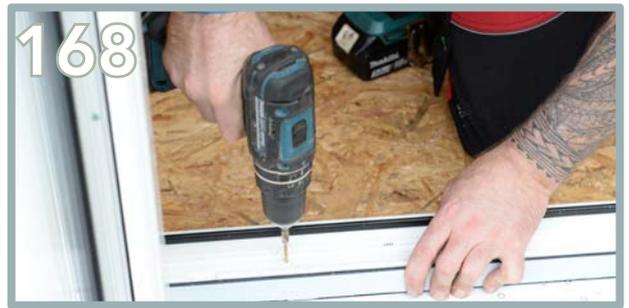
Drill 150mm from the both internal sides of the double doors. Use 112mm screws to screw into place at each side into the bottom of the frame as shown above.
