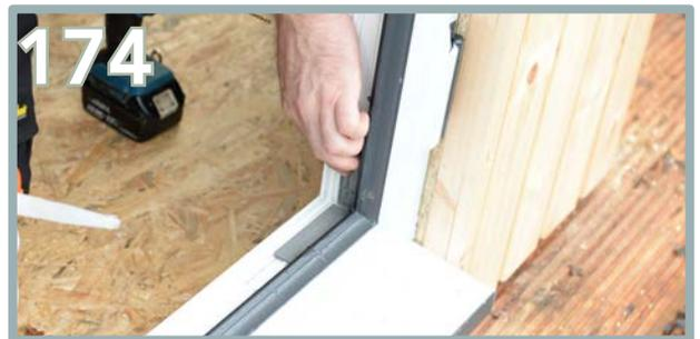
The glass should be packed using the toe and heel process. Toe and heeling works by supporting the double glazed unit with the packers.
