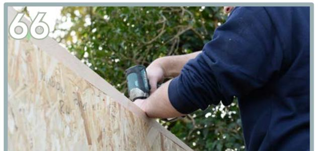
66 Use 2 x 35mm screws to secure the component within the thinner section. Repeat this process on the opposite side.
