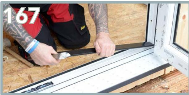
Remove the plastic strips from the bottom of the door frame. Keep hold of these pieces to re-apply afterwards.
