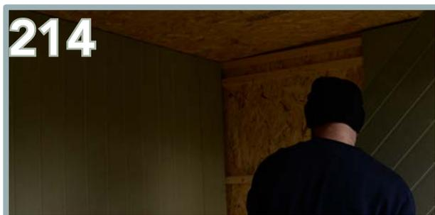
Butt up the next back panel with the rounded edge up against the chamfered edge and screw into place. There will be a trimmed board that will fit into the space. Use 8 x 50mm screws.
