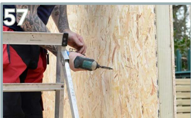
57 Internally position the screws each side of the adjoining split line. Use 5 x 35mm screws for each side of adjoining panels with the spline panel inside from top to bottom. Repeat this process for every adjoining panel.
