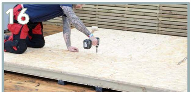
Screw the central screws into place, resulting in 3 in a row. This will result in 15 x 35mm screws per OSB sheet.
