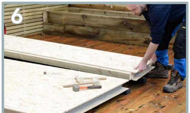
Place the second floor panel (A) onto the middle and end bearers. Ensure the panel is positioned half way on the middle bearer.
