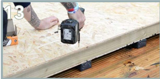
Pre-drill and use 4 x 125mm screws and ensure each screw goes into the bearer beneath. Screw 35mm screws in between the 125mm screws. Repeat process for the other floor capping.
