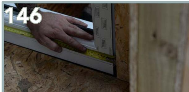
Apply adhesive silicone on to the base and carefully position the new frame into the aperture. Ensure to centralise it.
