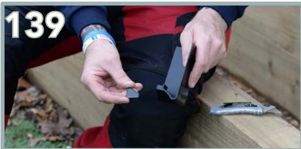
Simply break the excess off to produce the required gap as shown above.
