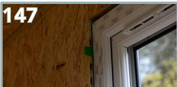
Insert packers underneath to level it and maintain the 5mm expansion gap. Ensure the back of the frame is in line with the OSB sheet inner face as shown above.
