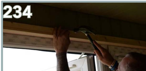
Fix into place using 6 x 30mm nails.
