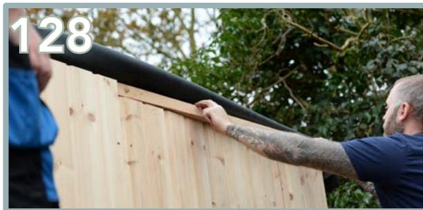
Before adding the plastic roof trims on the sides, the angled roof battens need to be applied to the gaps above the T&G panels. Fold the edge of the EPDM and slot in the batten onto the T&G side panel (BB).
