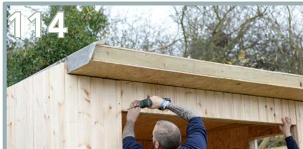
Apply the lintel panel (BL). This will fit in between the front panels. Use 6 x 80mm screws. Make sure to drill through the battens beneath.
