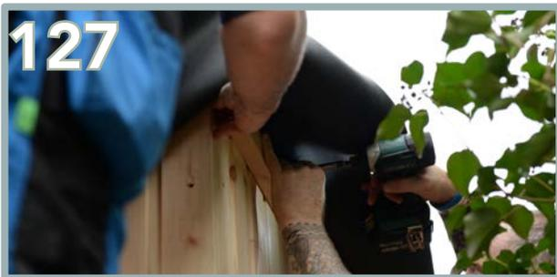
Underneath the EPDM, you will need to secure the back roof battens to the back T&G Panels (BM & BN). Ensure the battens edge is flush to the top of the T&G Panel. Secure with 3 x 80mm screws per batten.
