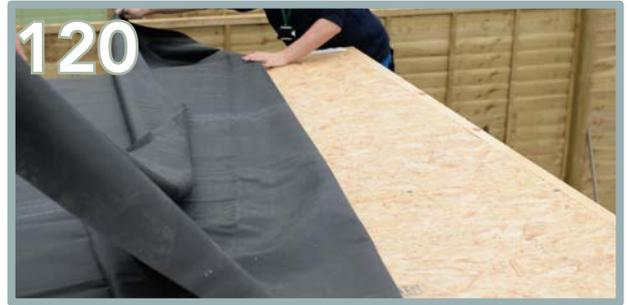
Fold the EPDM back to half way across the roof - we recommend two people for this. Be careful when moving on and around the roof to prevent any possible injuries.
