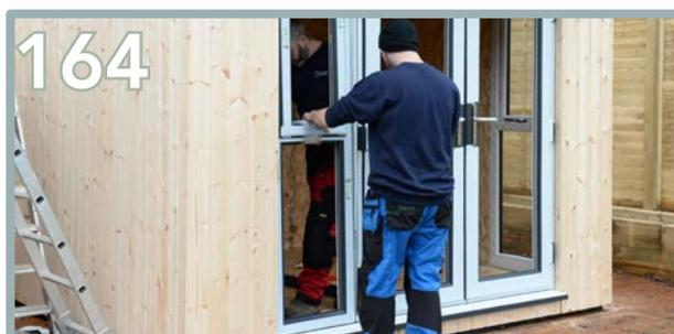
Insert the window frame into the left hand side of the double doors. The metal cap will slot into place.
