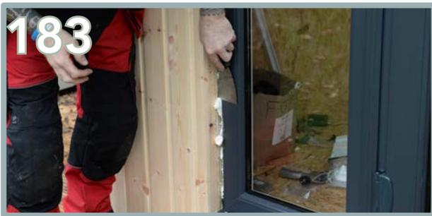
Remove all excess expanding foam around the window and door frames. Preferably it is better to wait for the expanding foam to cure before removing for easier removal.
