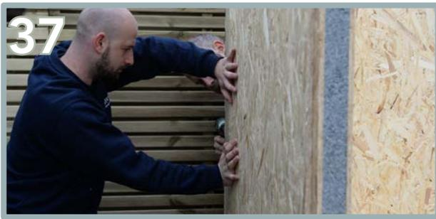
37 Add the expanding foam into the side groove of the Side Panel 1 (G) in the left back corner and butt it up against the first wall panel. Have one person holding onto the wall panel to prevent movement.
