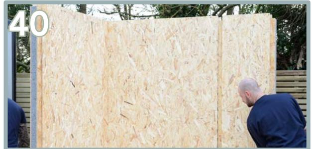
40 Slide the spline (Q) in the first panel (H). Please note that Xtend2.5 only has 2 x back panels.
