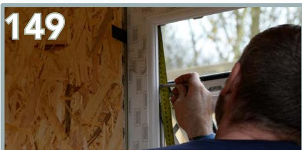
These should be drilled 150mm from the top and bottom corners and 300mm from the 150mm point at both sides. Use packers at the fixing points to avoid distortion to the frame.
