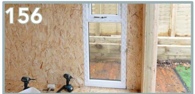
Repeat the same process for the bottom pane, ensuring it is centralised and packed properly with the toe and heel process.
