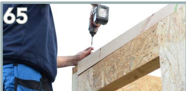
65 Use 2 x 125mm screws to secure the component within the thicker section.
