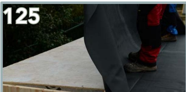
Continue with the glue application on the OSB roof surface as much as possible.
