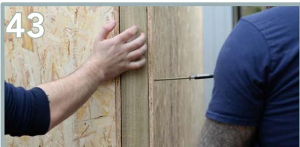
43 Pre-drill and screw through the back panel (H) into the side wall panel (G) using 3 x 150mm screws (top, middle and bottom).
