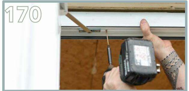
Repeat the process through the top. Drill 150mm from the both internal sides of the double doors. Use 112mm screws to screw through the top of the frame as shown above.
