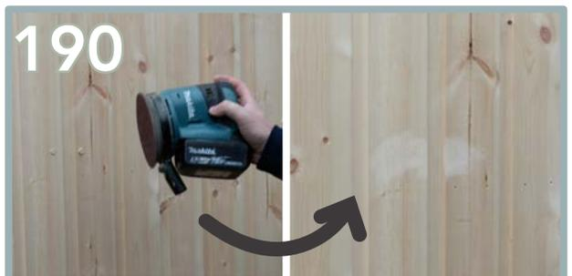
Finish with slightly cutting down and/or just sanding off any excess showing to produce a seamless finish. Repeat this process for every screw hole on the T&G panels.
