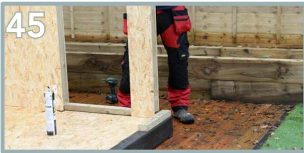
Apply the side wall panel (N1) as shown above, leaving the provided space for the window insert. This is labelled on the layout.
