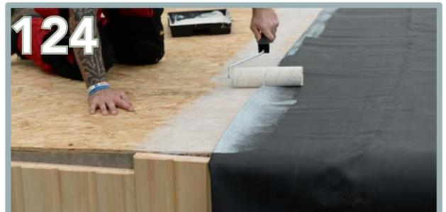
Repeat on the opposite half. Fold the EPDM back up until the point where the glue ended on the previous application.
