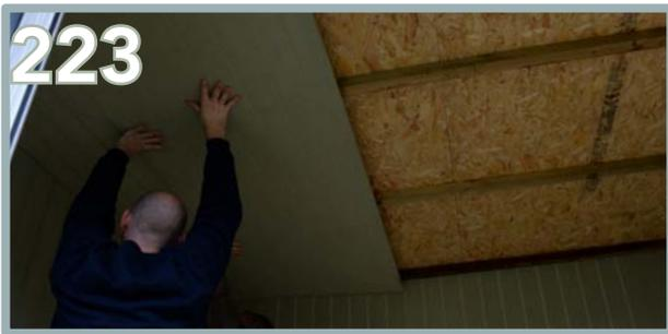
Start from the left side. Ensure the rounded edge is butted up against the side panels. You will need at least one person to hold the panel up whilst the other screws it into place.
