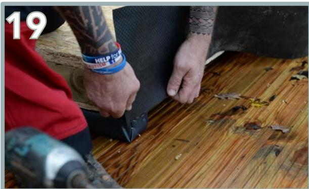
Start to unwrap the DPC roll and choose a starting point on the base's outer face. Ensure it covers half of the bearers and staple into place.
