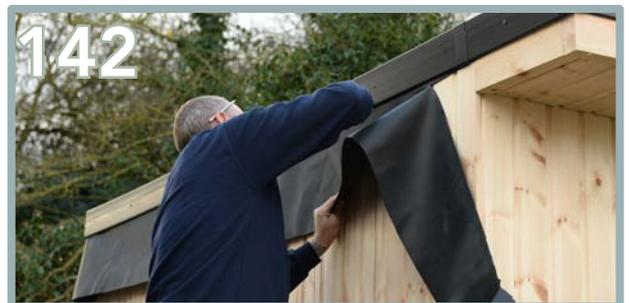
Once the plastic trims are complete around the roof, using a Stanley knife remove all of the EPDM excess. Use the plastic trims as a guide. Be careful not to cut the T&G panels behind.
