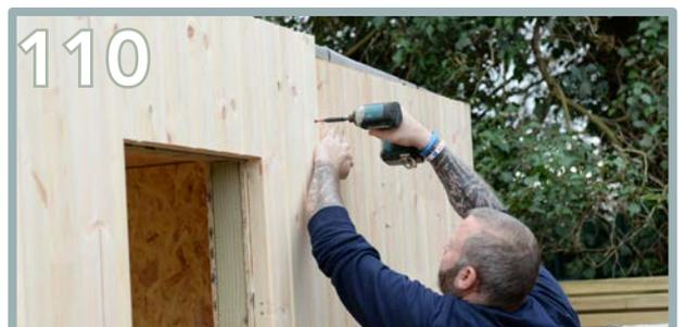
Ensure the opening of the cladding is flush around all edges to the window opening provided (BC). If not aligned properly, this will cause issues during the window installation.
