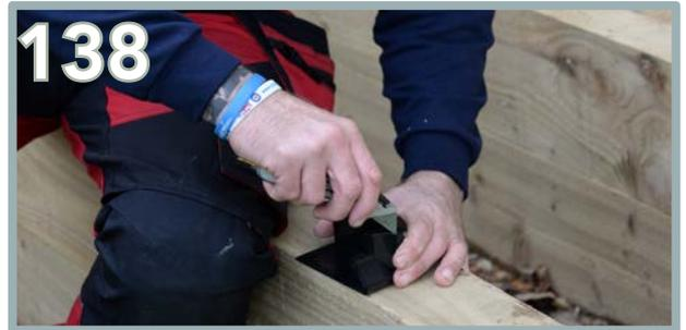
Before applying the corners onto the trims, you need to remove the plastic support. Use a Stanley knife to score an outline to weaken the support.
