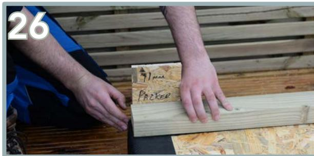
Starting with the back floor plate (AL), ensure it's flush end to end and provide 11mm spacing from the bases' back edge. Pre-drill and screw 4 x 125mm screws along the timber.
