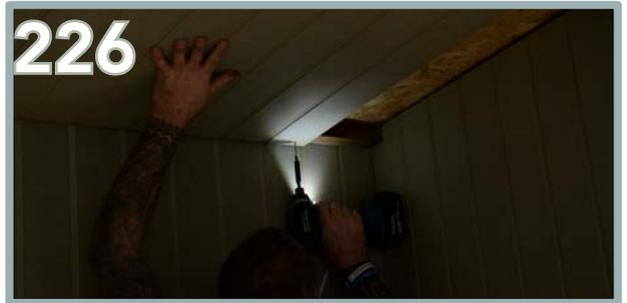
Use 4 x 50mm screws on each side and 2 x 50mm screws in the centre for both panels.
