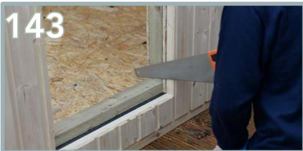
Remove the timber excess from the window section before inserting the window frame. Take out any screws in this section and cut with a saw, using the inner edge as a guide.
