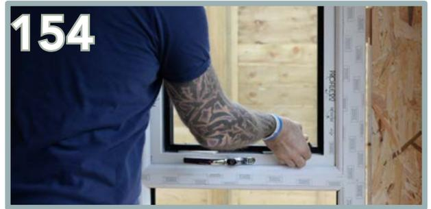
Place the top pane into position, ensuring it is centralised and packed correctly, holding the pane square.
