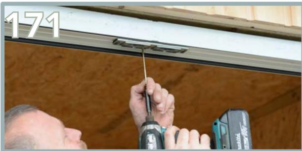
Repeat the same process centrally. Screw 1 x 112mm screw in the centre.
