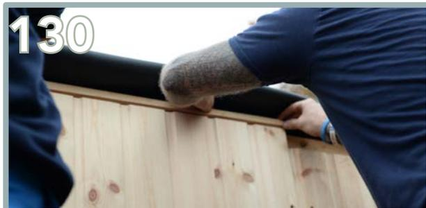
Repeat the same process for the smaller batten on top of the taller T&G side panel (BC) & (BA). Screw into place using 2 x 80mm screws. Repeat the process on the opposite side.
