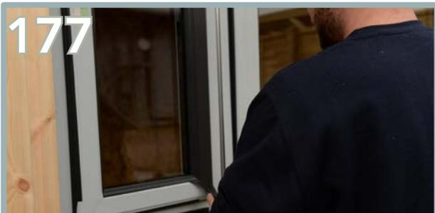
Repeat the same process for the other door and window panes, ensuring it is centralised and packed properly with the toe and heel process. Then add the window handle inside.
