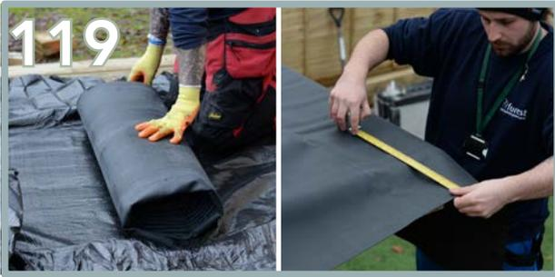
Unwrap the EPDM out onto the floor first, then measure out on the roof to ensure an equal overhang around all edges.
