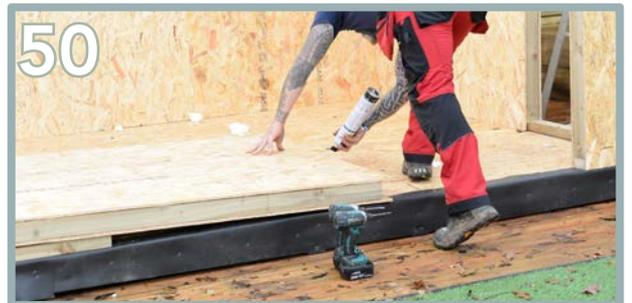
Apply the last left hand side panel (J). Apply expanding foam into the bottom groove.
