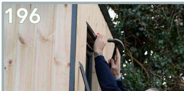
196 The same process applies for the window frame. Pre-drill and use 2 x pins on the front edge and 3 x pins underneath.
