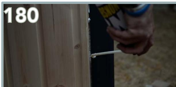
Apply expanding foam around the outer edge of the window frame.
