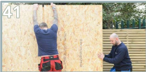
41 Add expanding foam into the inner side groove and into the bottom groove of the second back panel (H) and knock into place to complete the back wall.
