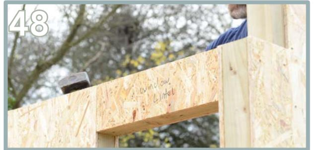
Knock the window insert (AA) into the section provided. Ensure the top is flush.
