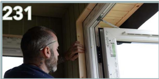
Apply the internal sides on either side of the door. Trim to fit if necessary. Use 5 x 60mm nails for each board to secure.
