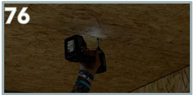
Pre-drill and screw 5 x 35mm screws, where the adjoining panels intersect.
