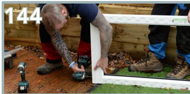
Remove any packaging from the new frame and screw the sill into the bottom of the frame. Use 2 x 50mm screws and ensure not to penetrate the inner skin of the frame.
