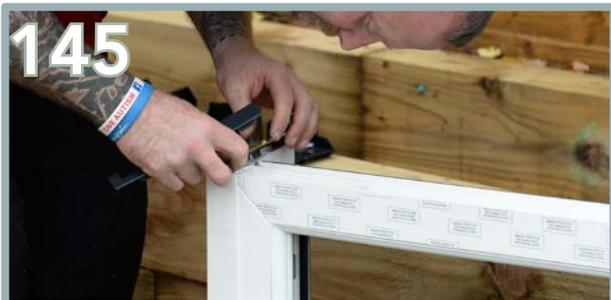
Be sure to seal the ends of sill with the caps provided to prevent moisture from tracking along into the wood work.
