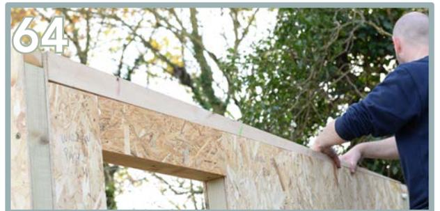
64 Position the furring (AB) and butt up against the front wall panel.
