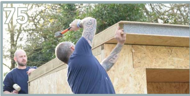
Knock further into place to allow the roof panel to be as flush as possible to the wall face.
