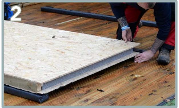
Place the first floor panel (B) on top of the two bearers and position it half way onto the second bearer. The black side covered in tar will be on top of the bearers as shown above.
