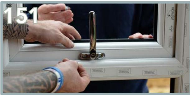
Apply the window handle with the screws provided. Remove the hole caps and drill the screws into the space provided. Then cover the holes back up with the caps.
