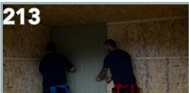
Start at the back left hand corner. Ensure the rounded edge of the panel is up against the wall. Use 4 x 50mm screws on each side and 2 x 50mm screws in the centre.
