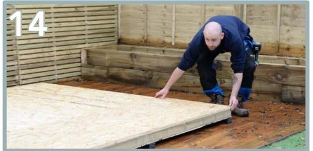
Apply OSB floor sheets (AG) on top of the SIPS panels one at a time. Ensure they are flush to all edges and screw into the corners to keep secure.
