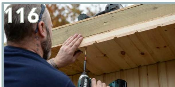
Apply the canopy panels (BJ) one at a time. Ensure they are flush to all edges. Apply 6 x 80mm screws per panel.
