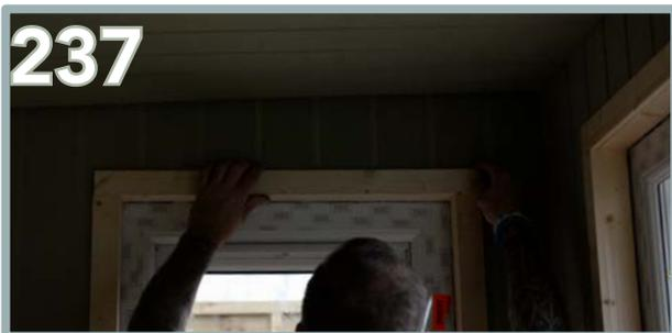
Apply the overlapping framing. Ensure flush around all edges and trim if necessary.
