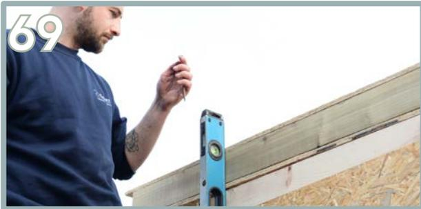
Use the spirit guide as a reference to screw through the roof panel into the side wall beneath. **Top Tip - Use the canopy T&G panel (BJ) as a reference for the correct overhang size.**
