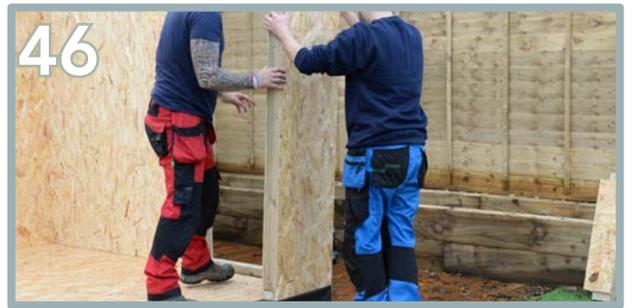
Apply the front wall panel (O) and butt up against the front side wall panel just secured. Ensure all edges are flush.
