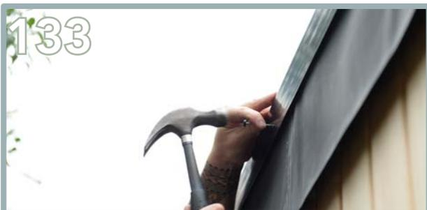
Use the pins provided with the plastic trims. Pin into the batten behind to secure in place.
