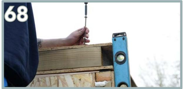
Position the back of the roof panel. Using the spirit level as a guide, the top OSB sheet on the roof panel needs to be flush to the back edge. Use 4 x 150mm screws along the edge.
