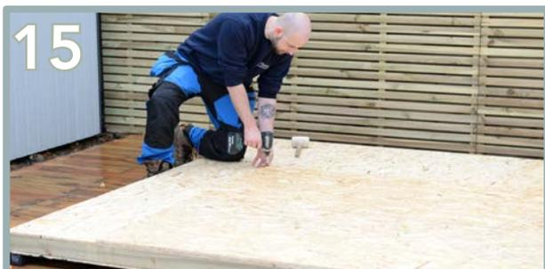
Using 35mm screws, screw 3 across the top and 5 down the sides of each OSB sheet. Screw along the edges first.
