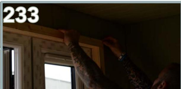
The top frame will sit on top of the side boards. Ensure both ends are flush to the side framing edge. Trim if necessary.
