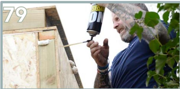
Use expanding foam in the roof panels groove across all 3 panels.
