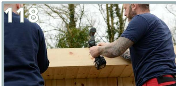
Position the front fascia. Ensure it is flush to the top and to the side fascia's outer face. Use 3 x 80mm screws centrally across the fascia. Repeat this process for the other front fascia.
