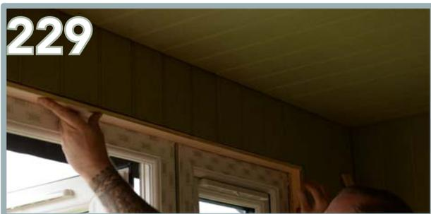
Start to apply the internal framing for the door. This is the same process as the external framing application. Start at the top, ensuring the board is flush to the edge.
