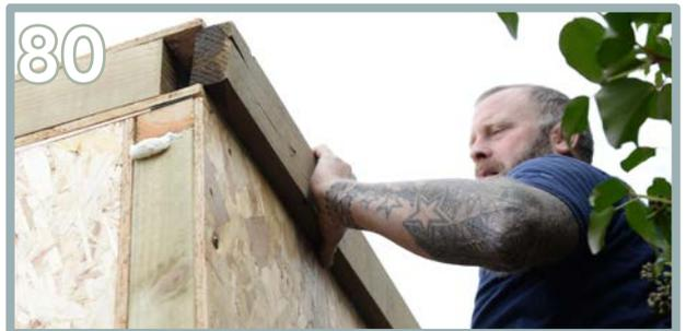
Insert the roof panel cap (AQ). Use 4 x 125mm screws through the panel cap and into the wall panel. Use 3 x 35mm screws, in between the 125mm screws to fully secure.
