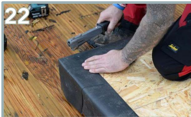
Using a Stanley knife, cut the DPC at the corner to create 2 pieces to easily fold onto the OSB sheets and staple into place.
