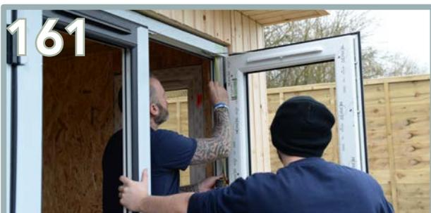
Check that frame is both level and plumb, then drill fixing holes into the frame side.
