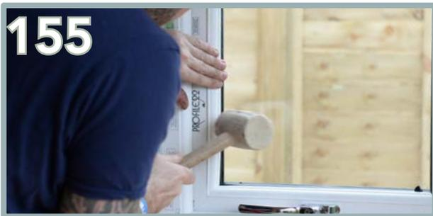
As the pane is positioned, the beading can be installed using a smaller rubber mallet and tapped securely back into place. Be careful to not aim at the glass pane.
