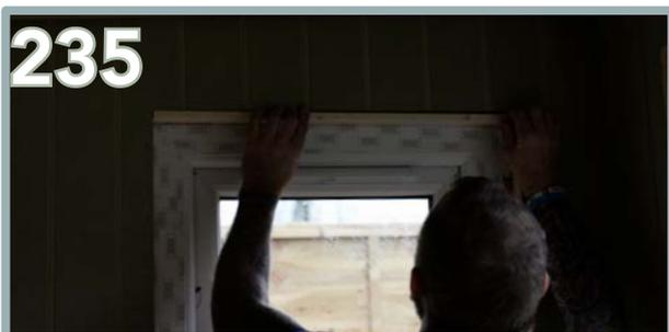
Repeat the same process for the window framing. Use 4 x 30mm nails to secure.
