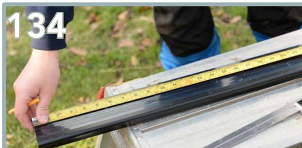
The other plastic trims will need to be measured out and cut using a hand saw to fit next to the fixed roof trim. Further detail will be shown throughout the application of the trims below.
