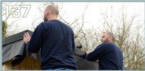
Measure and cut the plastic trims into 2 equal pieces. Ensure each end meets the side trims. Pin these into place. Add the clip in the centre of the adjoining trims.
