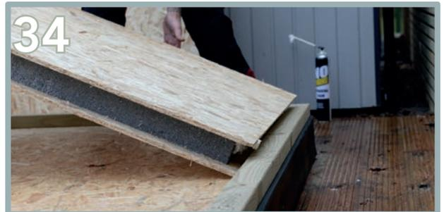
Begin the build at the left back corner, starting with Side Panel 2 (H). Insert the expanding foam provided into the bottom groove.
