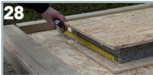
Pre-drill and use 4 x 125mm screws for the front floor plate (AL) Apply 2 x 125mm screws per end. Measure out your front panel (O) and ensure your front panel is placed flush to the edge.
