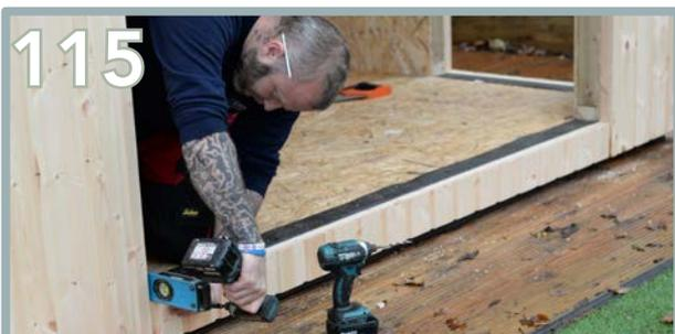
Repeat the same process as the lintel for the kick plate panel (BK) that goes underneath the door opening.
