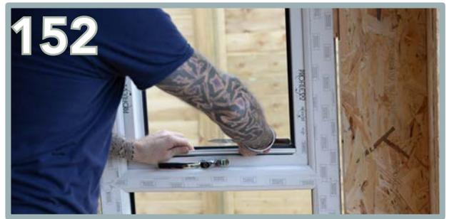
Using a chisel, break off the excess ends of the packers to create a neat finish. Remove the beading around the edge, ready for the glazing to be inserted.
