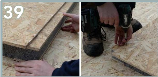
39 There will be smaller Spline panels (Q) that will be in between the grooves of some panels. Add expanding foam into each groove of the spline panel and apply them accordingly to the wall panel layout. Secure with 5 x 35mm screws.
