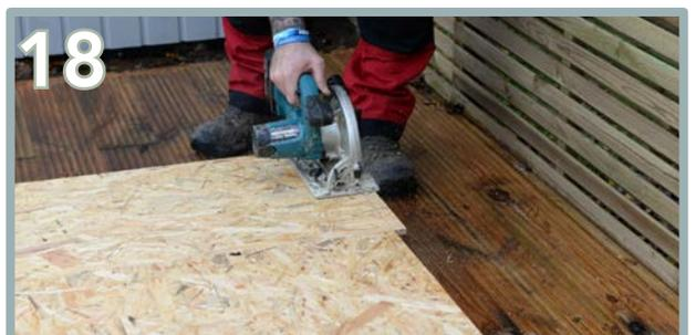
Some pieces may be oversized. If this is the case, saw the excess off after the piece is screwed into place, to create a flush finish.
