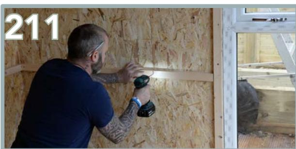
Apply the three shorter 45x28mm battens in between the window and back. These will be flush end to end and ensure they are the same height as the positioned back panels.
