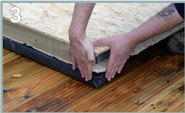
Ensure the panel is flush around the edges to the first bearer. Ensure the floor panels on the bearers are level using a spirit level as a guide.
