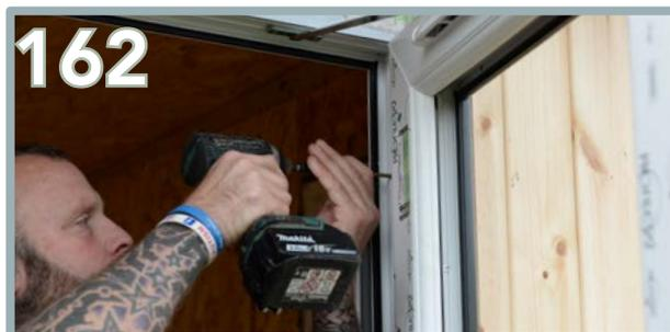
These should be drilled 150mm from the top and bottom corners and 300mm from the 150mm points with the 112mm screws.
