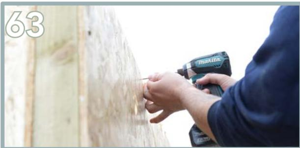
63 Further secure each all of the wall plates with 3 x 35mm screws externally and internally, through the OSB into the plate, in between the 125mm screws.
