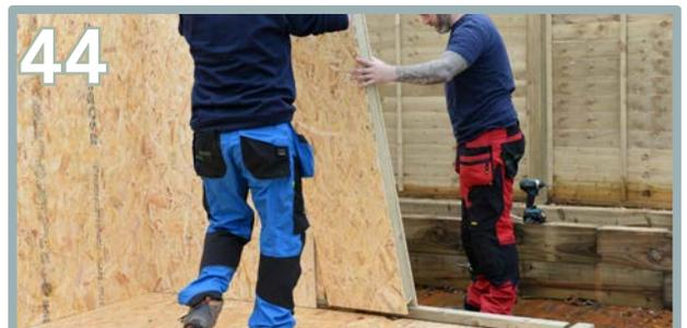
44 Continue on the right hand side panels as shown above (N), adding the expanding foam into the bottom grooves. Place and knock into the other side panel.
