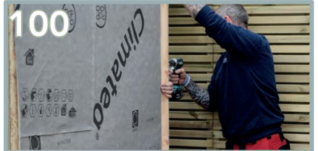
At each side, there will be a slight overhang of the T&G board. The battens edge underneath should be flush to the end. Use the 45 x 28mm batten as a guide to leave 45mm from the ground.
