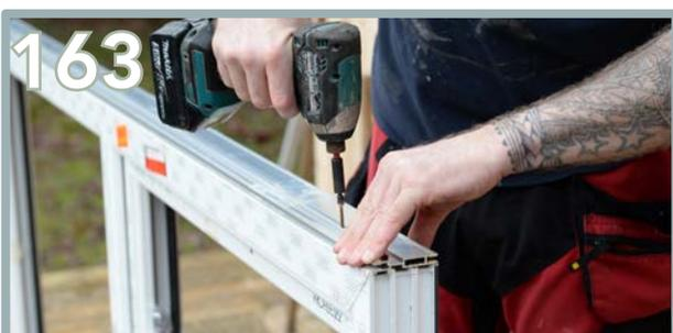
(This section is only for the 'Xtend Plus' doors and side window. This step will not apply to the standard option). Use 3 x 35mm screws to secure the metal capping.
