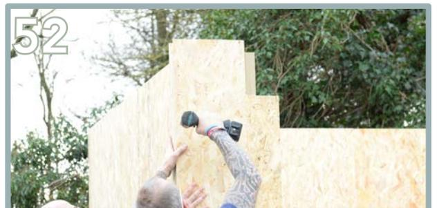
Apply the other front wall panel (O). Pre-drill and screw through the front into the side wall panel using 3 x 150mm screws (top, middle and bottom).
