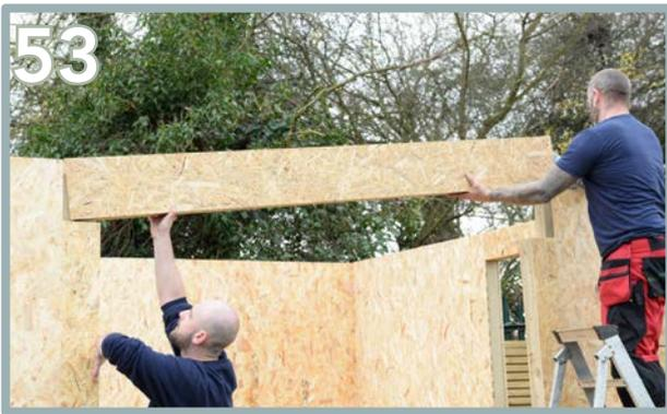
53 Insert the lintel piece (R) and knock into place. Ensure it is flush on the top.
