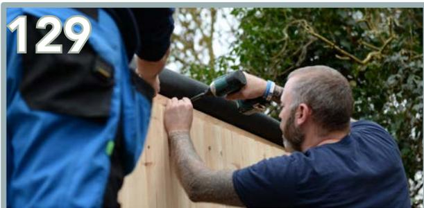
Screw into place using 2 x 80mm screws. Ensure the batten is butted up to the T&G panel and wall panel behind.
