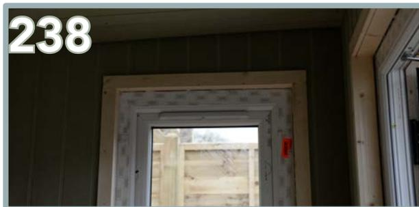
Use 5 x 30mm nails per side 45mm board. Finish with the top board using 4 x 30mm nails to secure.
