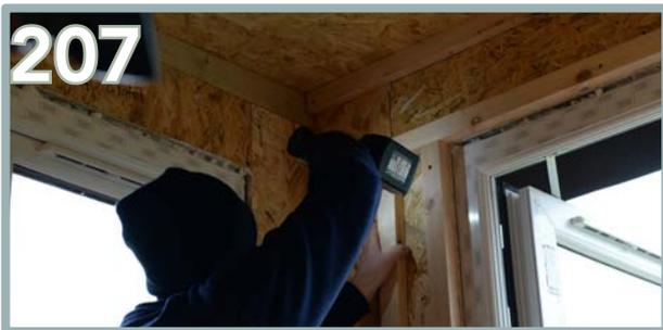
Then apply a batten in between the other two. Use 4 x 80mm screws and repeat on the opposite side of the door.
