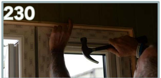
Nail into place using 6 x 30mm nails.
