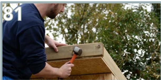
Use expanding foam and knock the roof panel cap (AQ) into place. Repeat the same process. Ensure they are flush to all edges.
