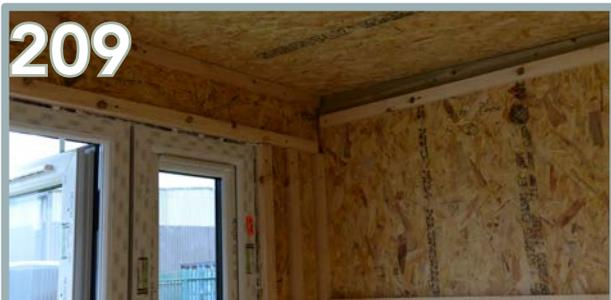
Use 5 x 80mm screws for each batten. The battens on the left hand side will not be aligned to the front batten positions.
