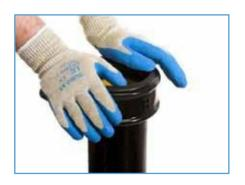
3. . Push the socket over the end of the pipe after lubricating both pipe and gasket ensuring the pipe end is fully inserted and abutting the central regis ter in the socket.
