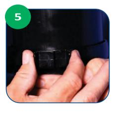
\* Squeeze the clips at the back together to secure the Strapon Boss to the soil pipe.
