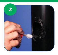
\* Solvent weld around the hole and the flange of the Strap on Boss.
