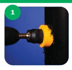
\* Cut a 54mm hole into the soil pipe.
