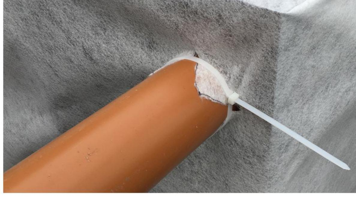
Wrap all outward faces of the installation in geotextile membrane. Cut the membrane where the pipe meets the crate, peel it back and secure it around the pipe with a large cable tie (included in our cubic metre sets).
